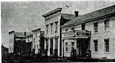
The Guy House, built in 1868 on the N.W. corner of Main and Black. Later it became the Northern Pacific Hotel.
