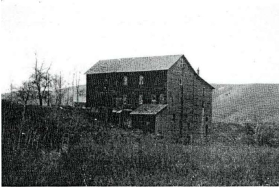
THE COVER FLOUR MILL AT BOZEMAN Built in 1865 by Tom Cover and Perry (Bud) McAdow. Courtesy, Montana Historical Society
